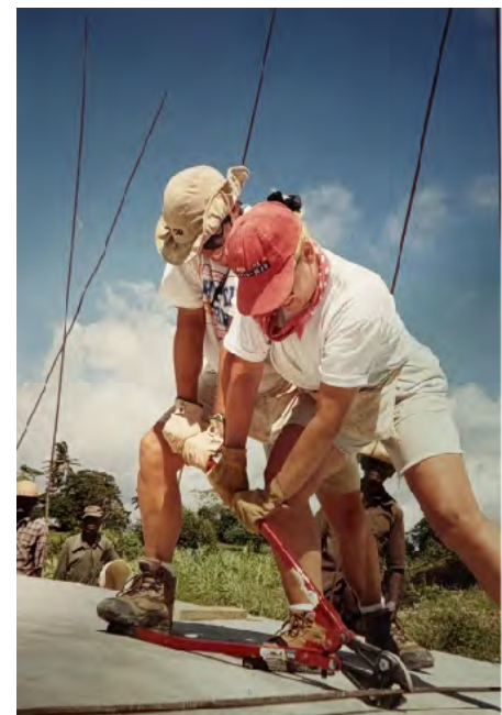
Ann and volunteer cutting rebar
